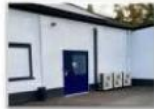
Back View & Entrance
